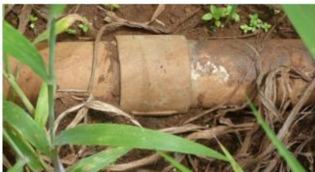
Proper pipe connection
