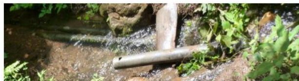
Due to the leakage, the overflow was tremendous, and much water was wasted.
